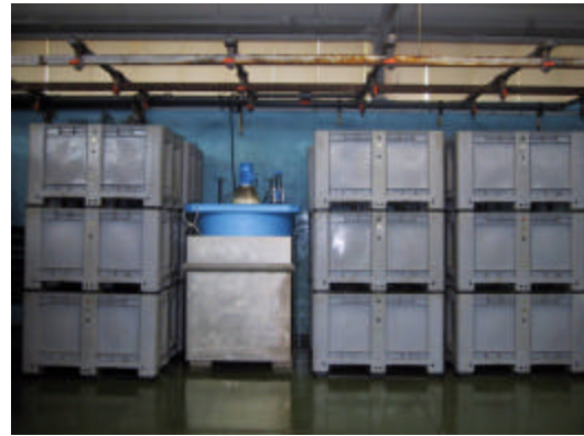
Skim in small Tank (sump) together with bins
